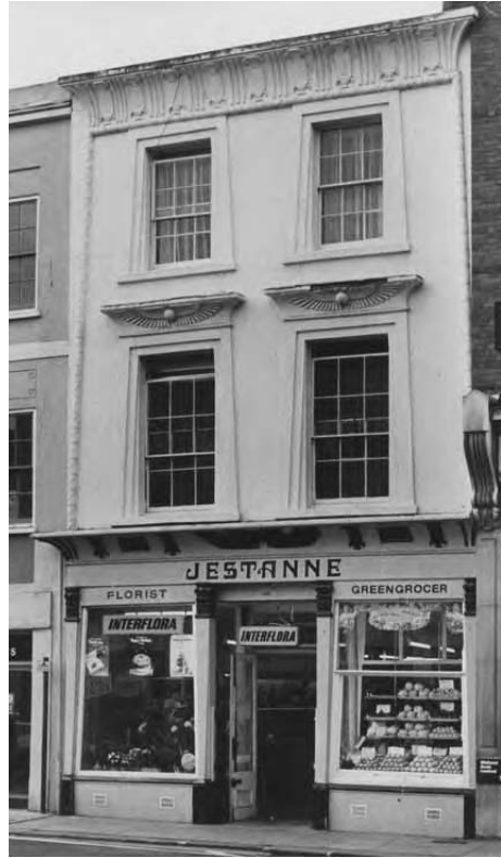
Plate 157 No. 42 Fore Street, Hertford: a remarkable survival, with shop-front in the Egyptian style, and a street-front above with battered Egyptianising architraves. Photograph of 1978 (JSC).
